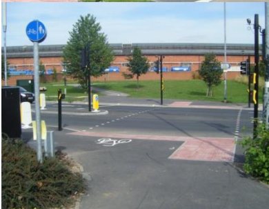
Toucan crossing (combined pedestrian and cycle crossing) - £40,000 - £50,000 - only appropriate where there are existing off road cycle facilities or they are being provided as part of a scheme.
